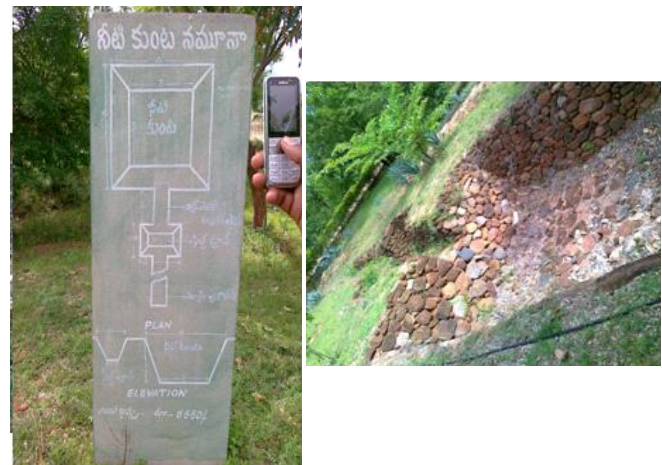
Mini percolation tank constructed by IWMP at Mahaboobnagar district in the fields of Ramesh
