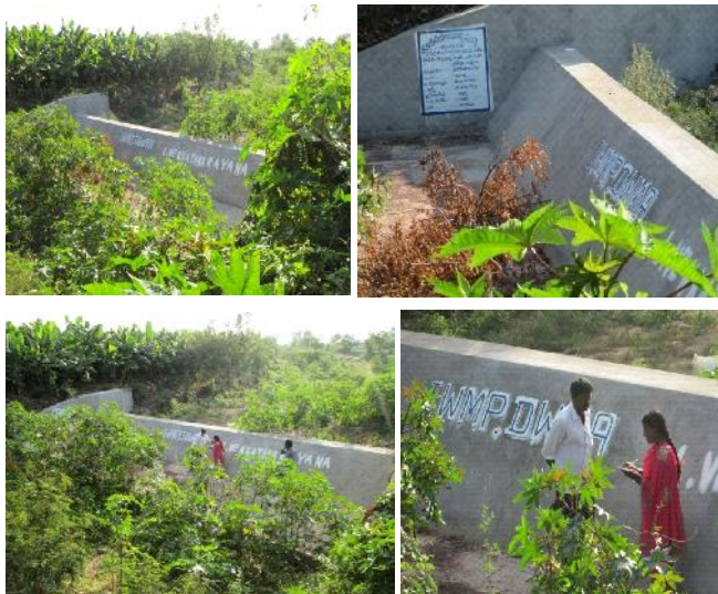
Check dam constructed by the IWMP at Ananthapur district in the fields of Venkatanarayana
