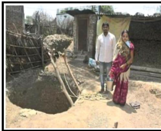
Excavation of 25 feet well by poor family during lockdown period
