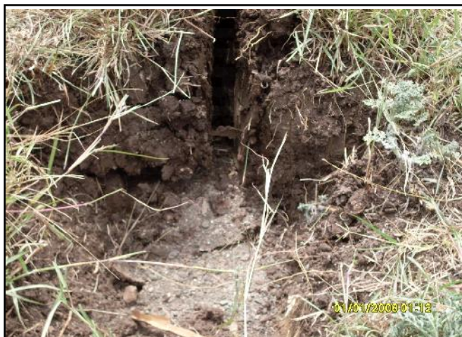
Fig. 3 : Success of mole formation and sand filling
