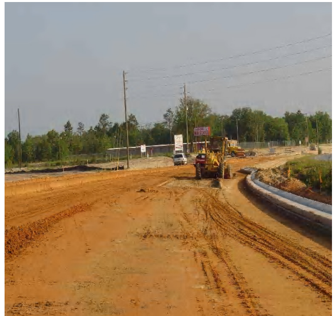
Fig. 2 : Sub-grade of N.H. 1
