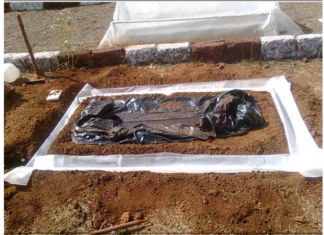
Plate B: Third channel from all bottom sides for W-shape solar still on ground
