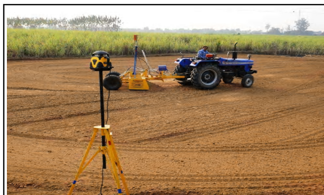
Fig. : Laser leveler in operation
