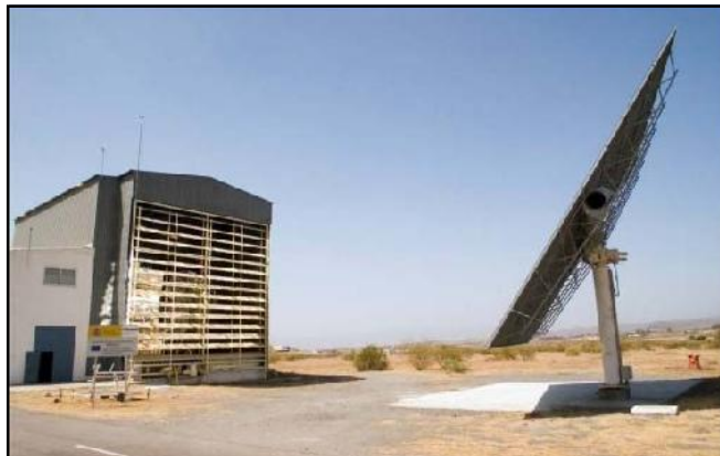
Fig. 4 : The 60 kW solar furnace at the PSA (Source: PSA)
