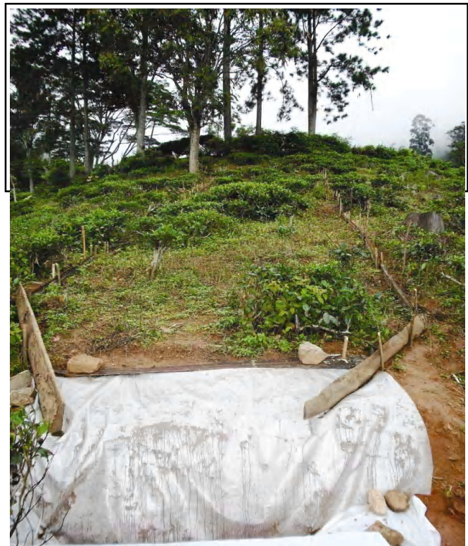
Fig. 1: Sedimentation pits which have been well covered using white durable polythene
