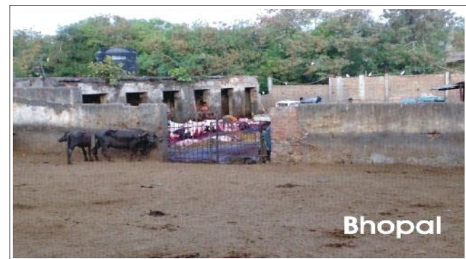
Fig. 6 : Indicating no lairage and compound facility
