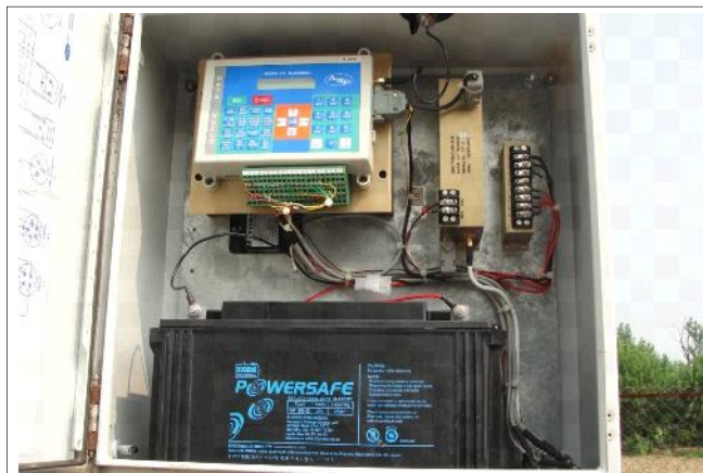
Fig. D : Data logger of automatic weather station
