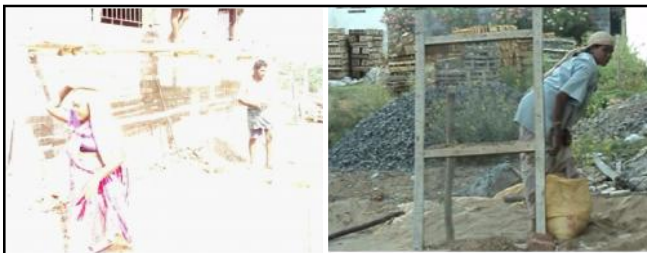
Fig. 2 : Working in summer and winter with difficulty
