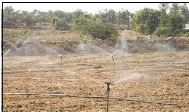
Fig. 3 : On field installation of sprinkler irrigation system
