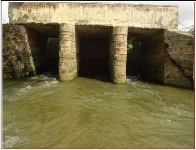
Fig. B : Regulators at the head reach of PT channel
